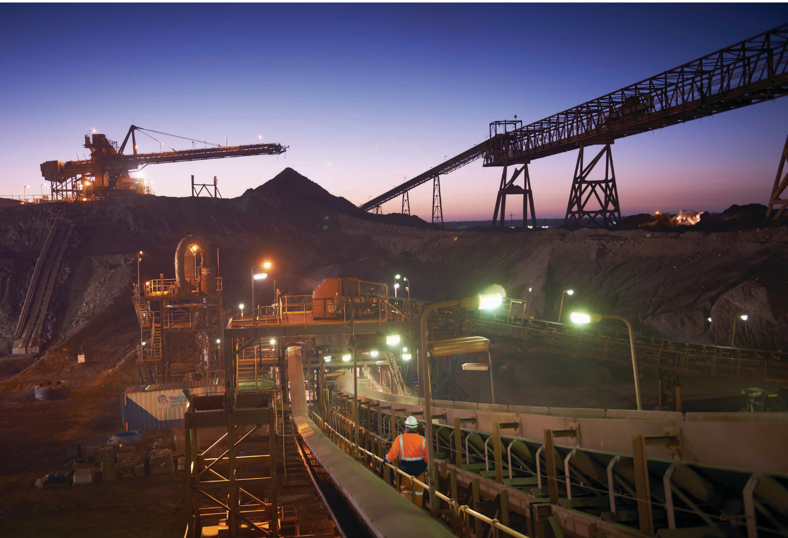
Dusk at the Olympic Dam processing plant. Source BHP.
