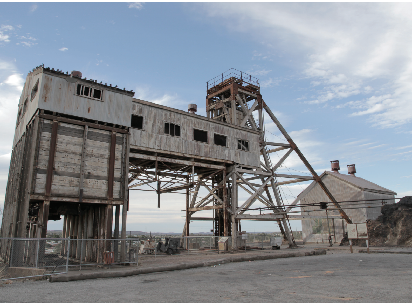
The 1890's wooden headframe erected over the Browne Shaft at the Broken Hill Junction Mine — one of the sites that will be visited during the pre-Convention Broken Hill fieldtrip. Photo courtesy of Jared Broome, Perilya Ltd.
